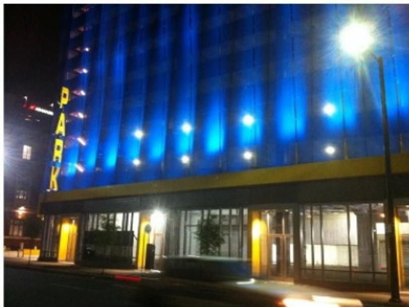
*ACTUAL PICTURE OF PARKING GARAGE*
