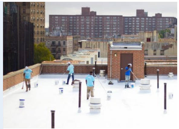
NYC CoolRoofs trainees coat a rooftop with white reflective paint.
