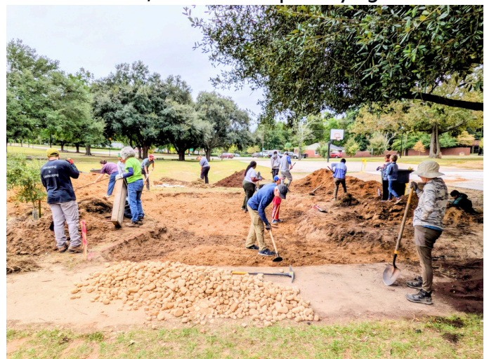
Rain Garden Installation in Columbia, SC (Gills Creek Watershed Association). October 2025.
