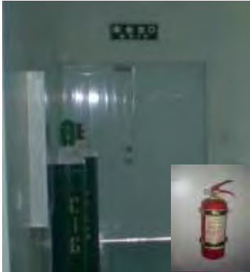
Exit sign in Chinese with door that lacks bolting mechanisms
