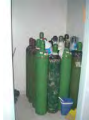
Unsecured oxygen tanks
