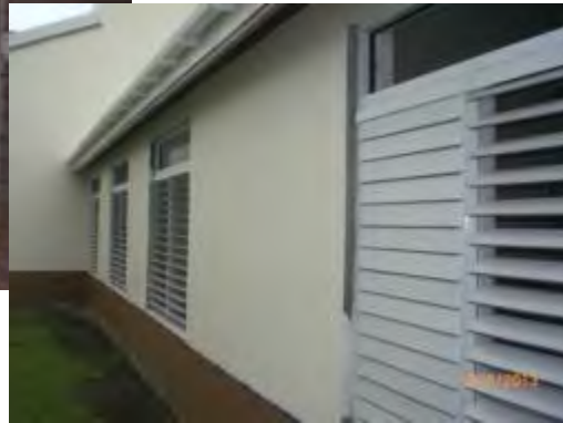
Aluminium windows installed above ground level and with transom for day lighting
