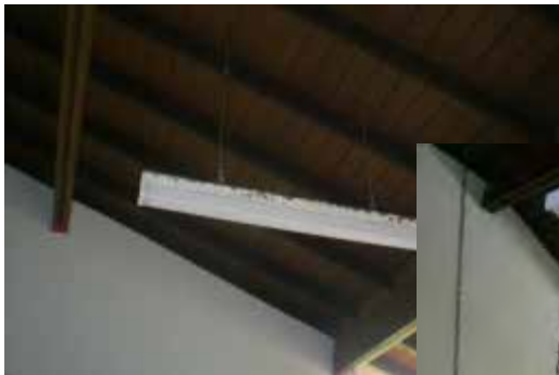
Old rusting tubular fluorescent light fixture
