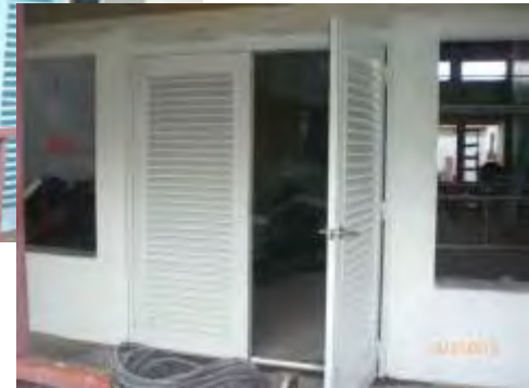
New, aluminium, hurricane resistant doors
