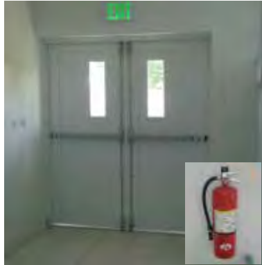
Large exit sign with new door with look through & crash bar mechanism
