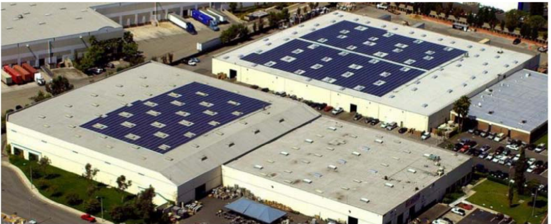
A 743 kilo-watt Solar System in City of Industry.
